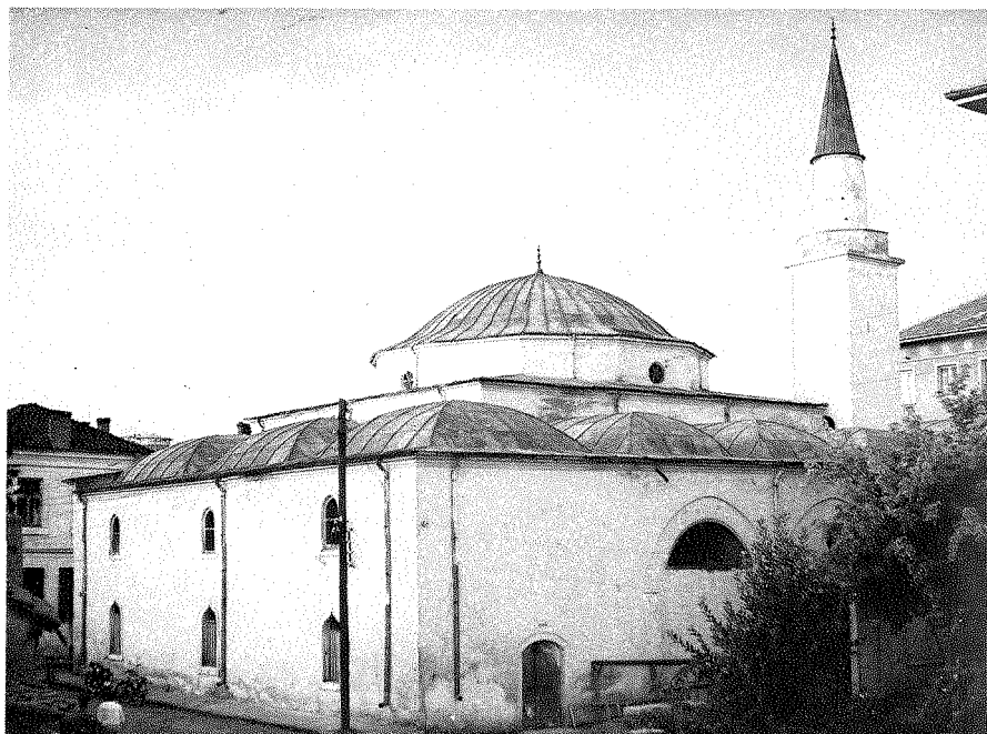
Fig. 9 — Jambol, Eski Camii. General view in 1970. Note the enclosed 'son cemaat yeri' and its walled-up arches. A small door has been made from a window.
